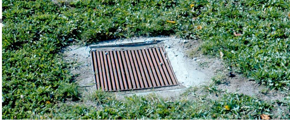
Catch basins are typically of open grate design and are usually installed on main drains.
